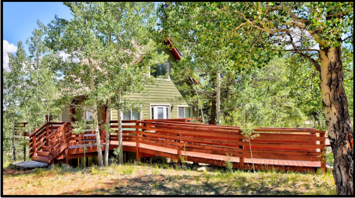
Figure 28: Defensible space around the Park’s existing structures should be monitored and maintained annually.
