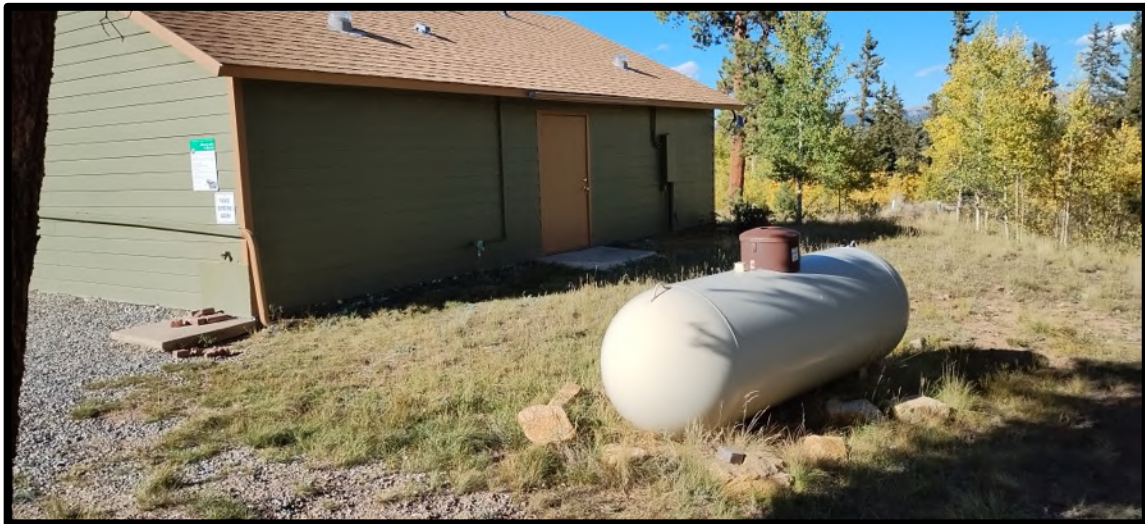
Figure 41: Keeping grasses around the Comfort Station and propane tank to 6 inches or less is highly recommended to maintain the defensible space that already exists. Adding a layer of gravel around the base of the propane tank that extends out a few feet on all sides would create a non-flammable perimeter that would help keep fuels like burning grasses from making direct contact with the tank during a wildfire event.
