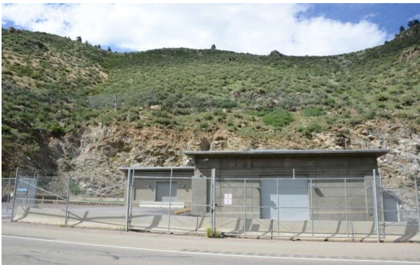
Roberts Tunnel Hwy 285 south of Grant
